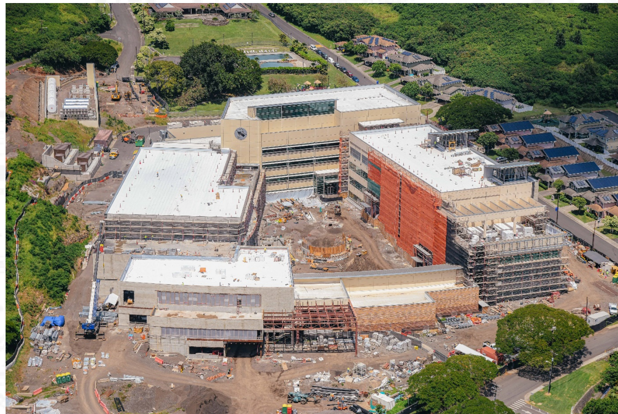
C2F under construction
