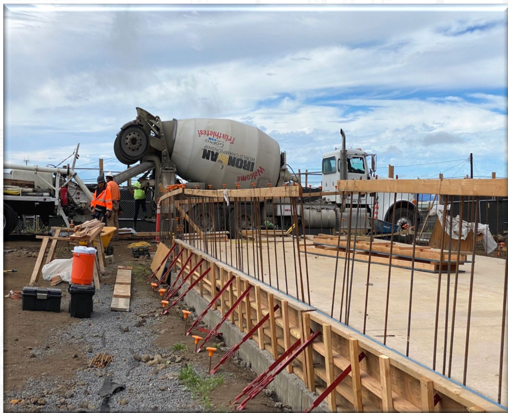
Construction at Pohakuloa Training Area
